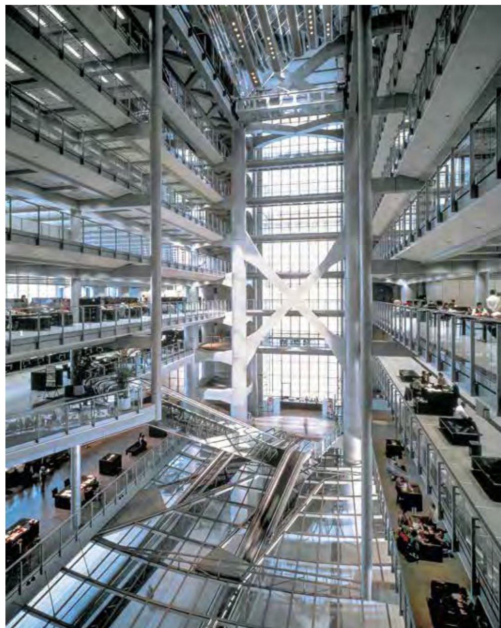
Hongkong and Shanghai Bank Headquarters, Hong Kong, China, 1979 – 1986, Looking into the atrium. Natural sunlight is the major source of lighting inside the building. There is a bank of giant mirrors at the top of the atrium, which can reflect natural sunlight into the atrium and down into the plaza.
